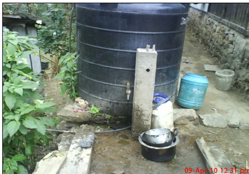
Photo Plate 9- Drinking Water Tap at Lethang Village
