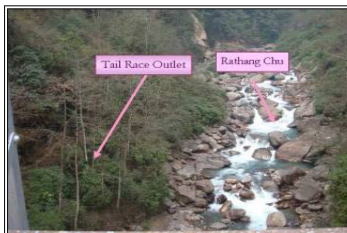
Photo Plate 2 - Lethang HEP – Tail Race Tunnel
