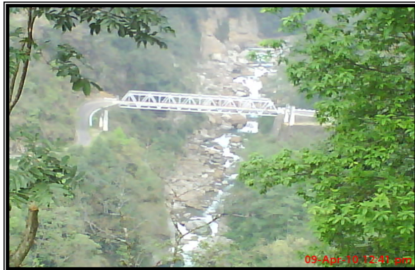
Photo Plate-6 -Lethang TRT Bridge Road connecting Yuksam
