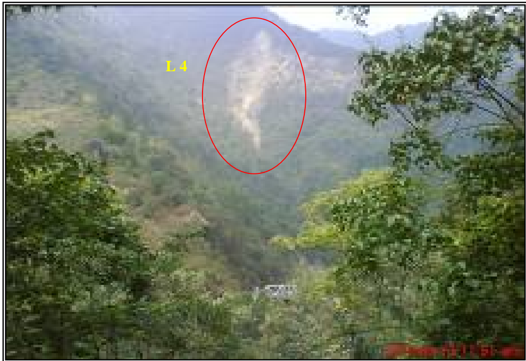
PhotoPlate-3 :Landslide area near TRT
